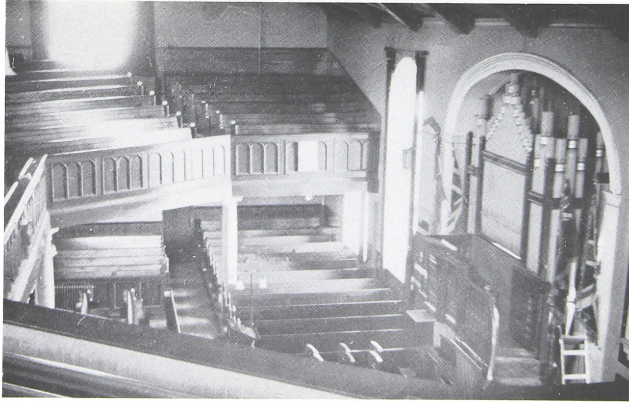
ELLON PARISH CHURCH: INTERIOR BEFORE RENOVATION
